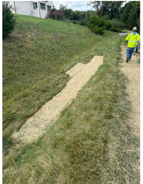
Natural Swale - After Maintenance
